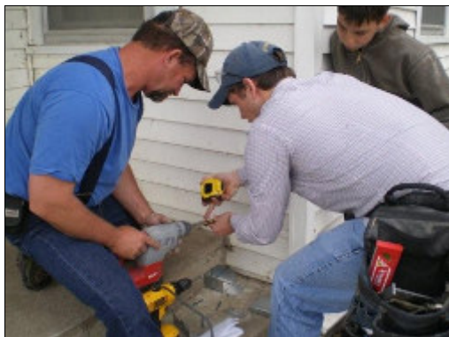
Our church is developing a mercy needs response ministry with other local churches. Our first project this year was to build a wheelchair ramp for a farmer's wife. Here, CTR church member Chris (foreground) shows our son Peter (right) and a member of another church how to anchor posts.
